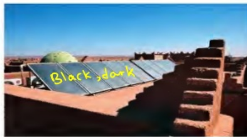
▲ Figure 15.12 Shiny and white surfaces reflect thermal radiation, while matt black surfaces, like in the solar heating panels, absorb it.
